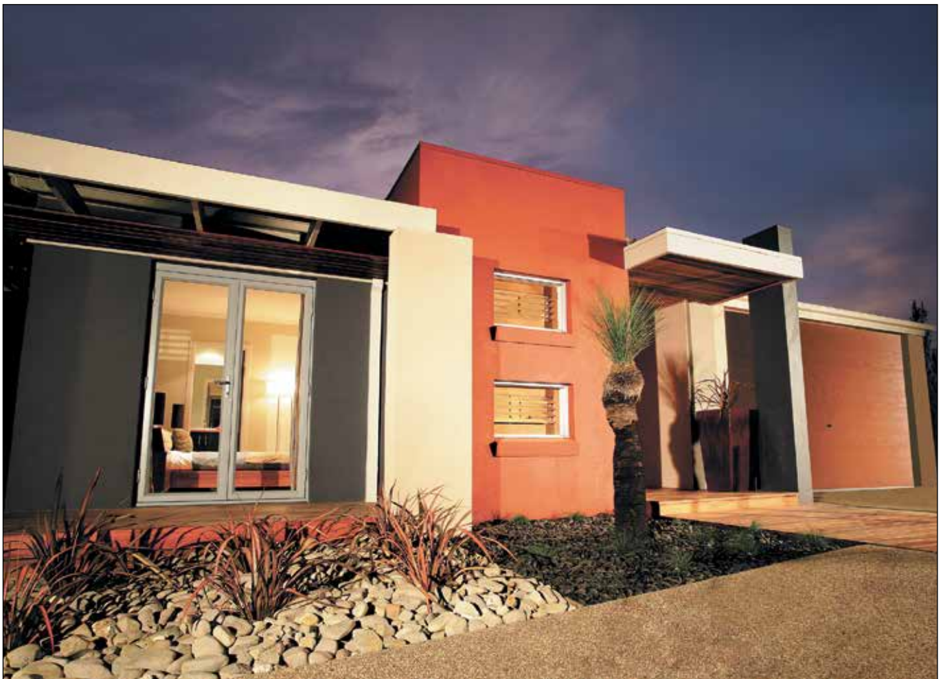
An example of a home built with Hebel. Photo courtesy of Metricon
