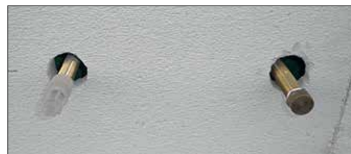
Fig. 3.3 – Neat Finishes of Installed Services
