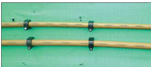
Fig. 3.2 – Installed Piping Services Prior to the Installation of Hebel PowerPanel XL
