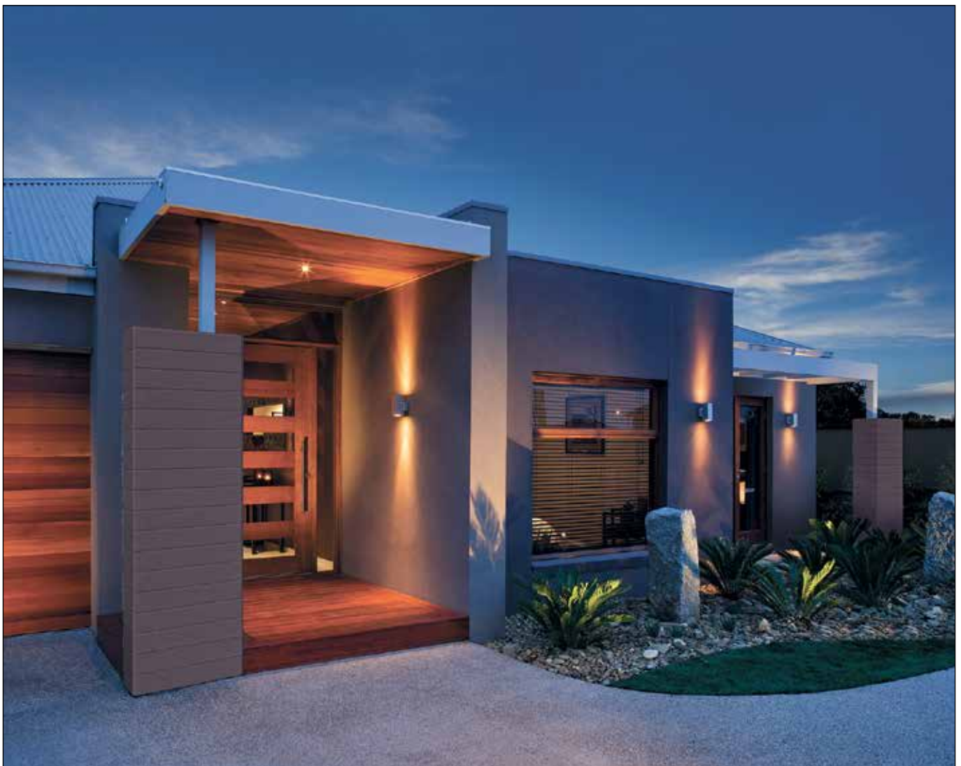
An example of a home built with Hebel. Photo courtesy of Metricon
